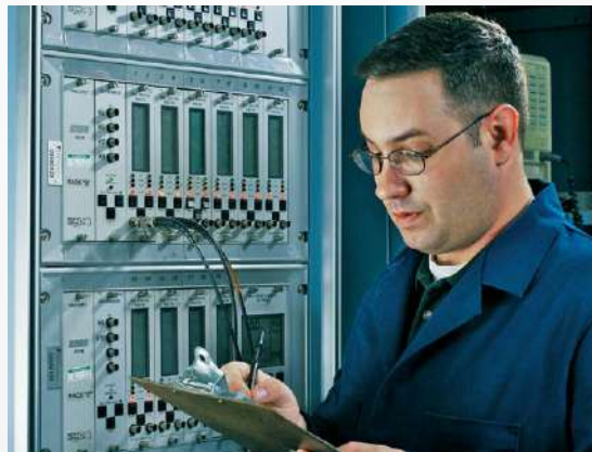
The test center control room provides computer control of cooling water, input speed and lubricating oil supply
